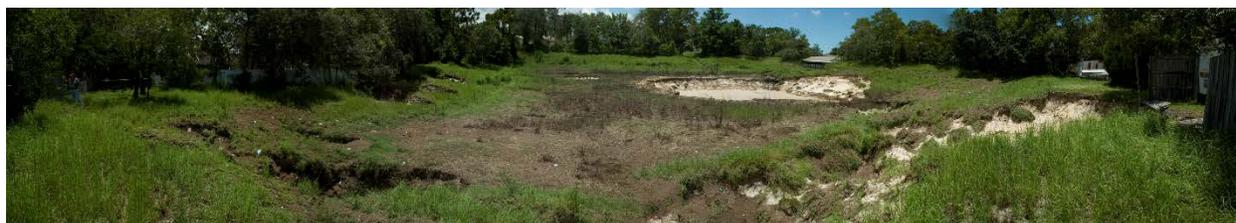
**Figure 5.** Sinkholes formed within and near this stormwater pond after Tropical Storm (TS) Debby in June 2012 in Spring Hill, Hernando County.
